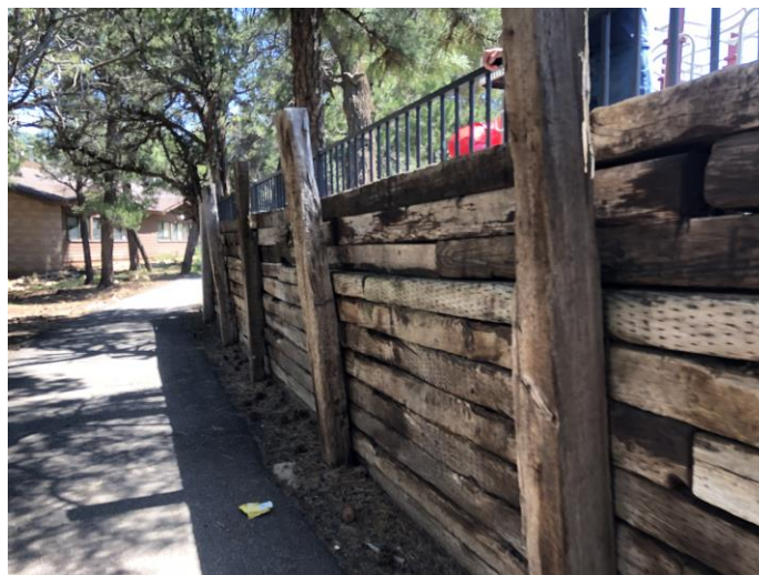
Figure 3: Current Retaining Wall at GCHS
